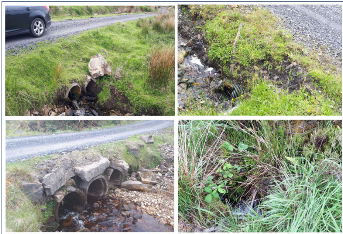
Photo 3: Examples of Pipe Culverts (Source, FT)
