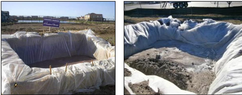
Plate 6-1 Typical concrete shoot wash out areas
