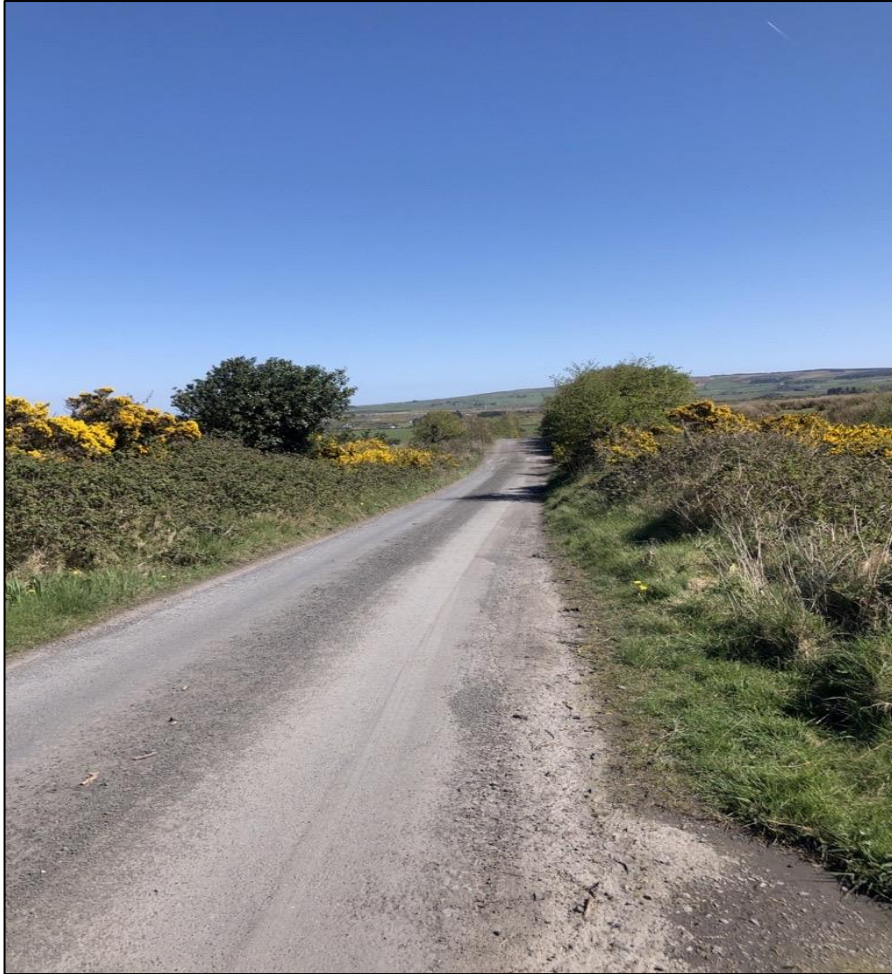
Plate 3-16 Existing Road (BL3) into which the cable is going to be laid.
