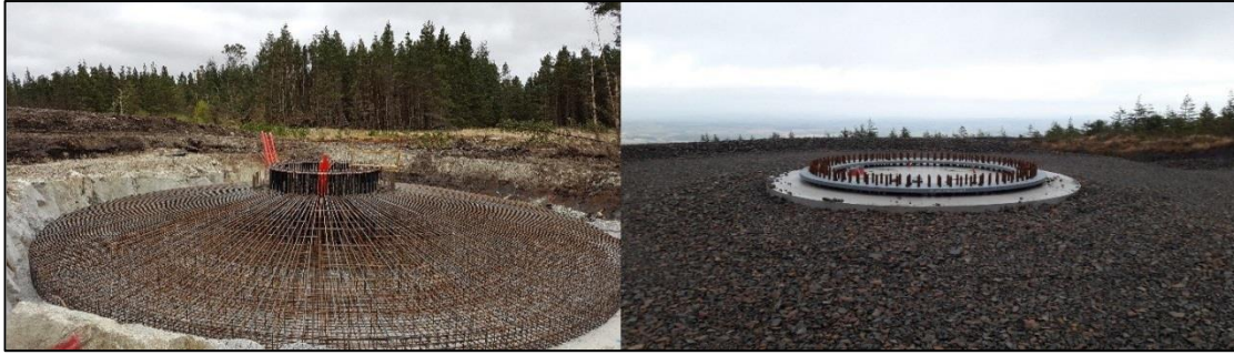
Plate 2-1 Turbine 'Anchor Cage' and Finished Turbine Base
